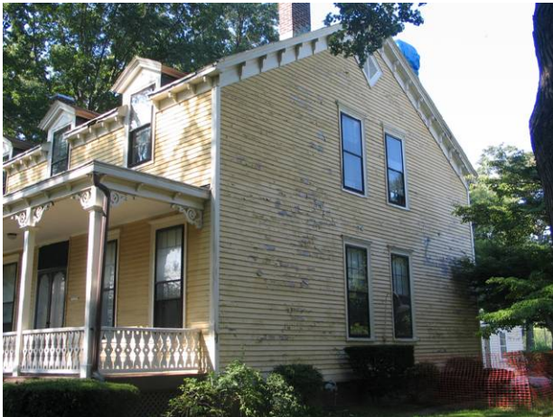
Nolan Park house before stabilization
