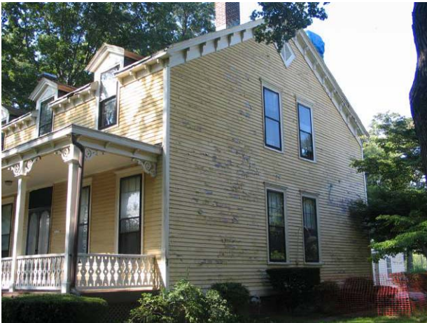
Nolan Park house before stabilization
